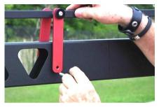
11. As you attach Parallel beams, use the swing arms to support the Beams. Space them differently depending on the length you are building the Crane.
