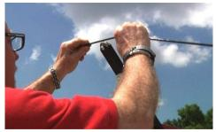
21. Pull the cable up to the top cable roller on the cable pole and lay the cable into the roller track. Do this to both the right and left sides.
